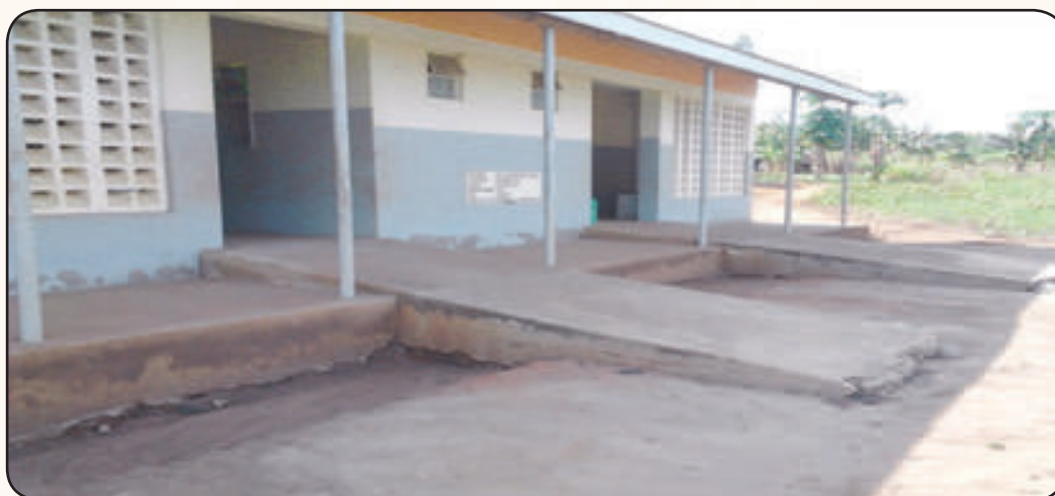
A ramp at Karuma HC II, Kiryandongo District that requires backfilling as a result of soil erosion
