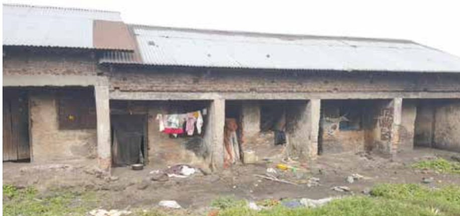
◀ One of the dilapidated structures where Batwa in Kisoro live
