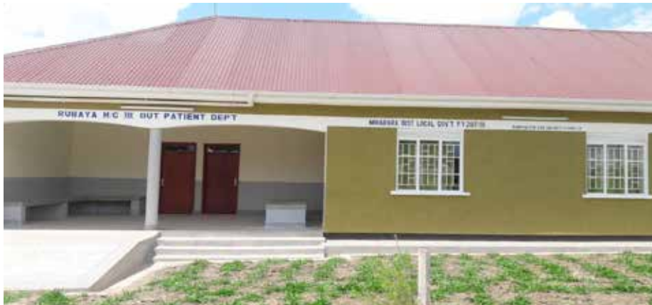
◀ Newly constructed structure at Rubaya Health Centre III in Mbarara district.
