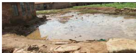
Houses/settlement in Bwaise I and III in Kampala flooded by rainwater ▲
