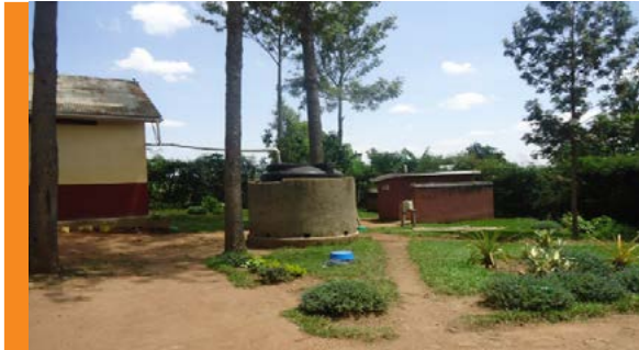
A rain-harvesting water tank at Butenga Prison in Bukomansimbi district
