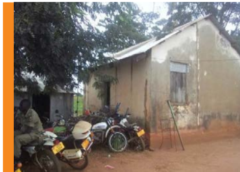
Building that houses Nwoya CPS.
