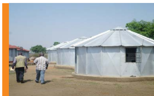
Newly constructed uniports at Ragem Prison in Nebbi district
