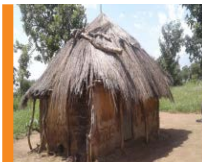
Police accommodation at Ogor Police post, June 2017
