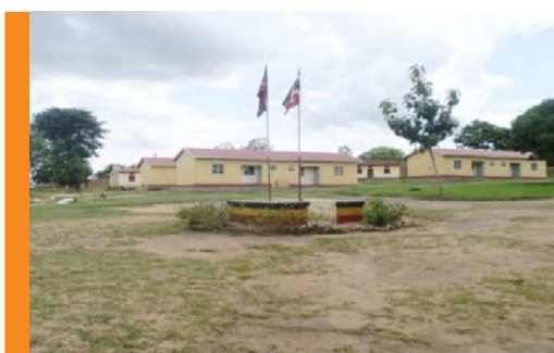
Staff quarters recently renovated at Koboko Prison
