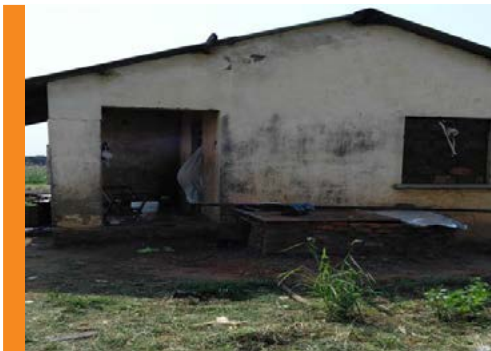
Building occupied by Lamwo CPS in Padibe
